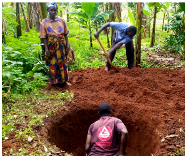
Above, a new pit latrine under way. Below, a completed latrine
