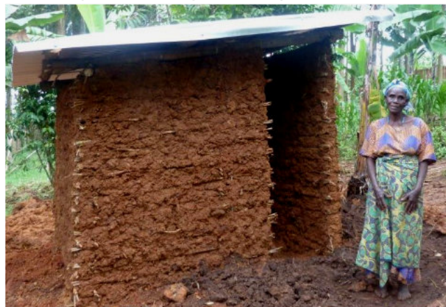
Above, a new pit latrine under way. Below, a completed latrine
